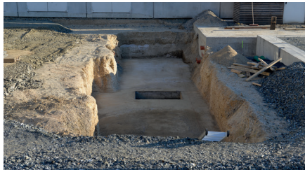
The base slab is concreted on site in accordance with specifications.
