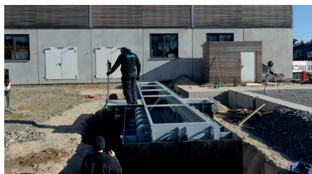
The TRUCKBAY is levelled before casting.
