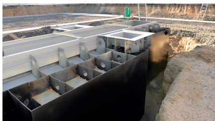
The double wall is now filled with concrete to achieve the required stability.
