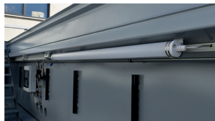
LED tube luminaire, 1630 mm long, 3800 lm
