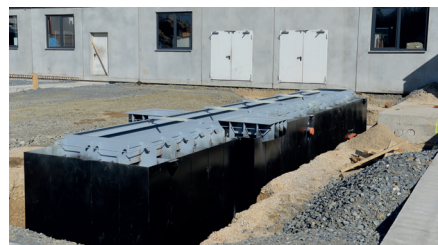
Once the concrete has set, the pit body can be cast in the floor.
